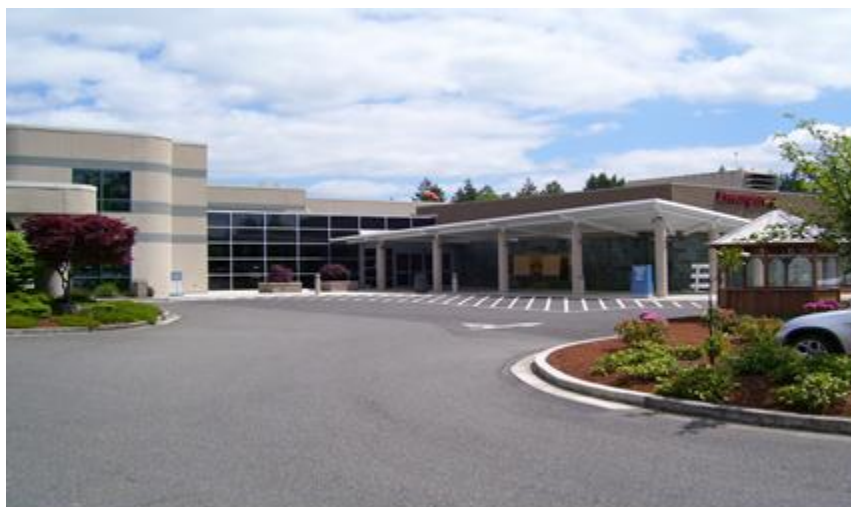
PROVIDENCE CENTRALIA HOSPITAL DIAGNOSTIC IMAGING DEPT – OFF SCHEUBER
